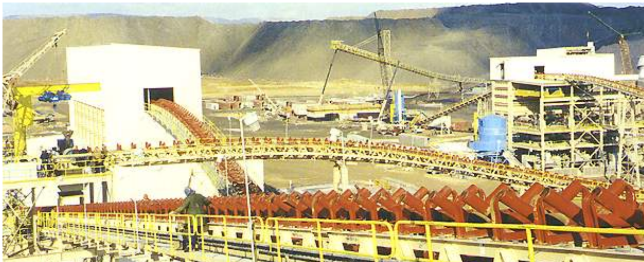
Newmont's Zarafshan mining complex (SPG Media Group)
